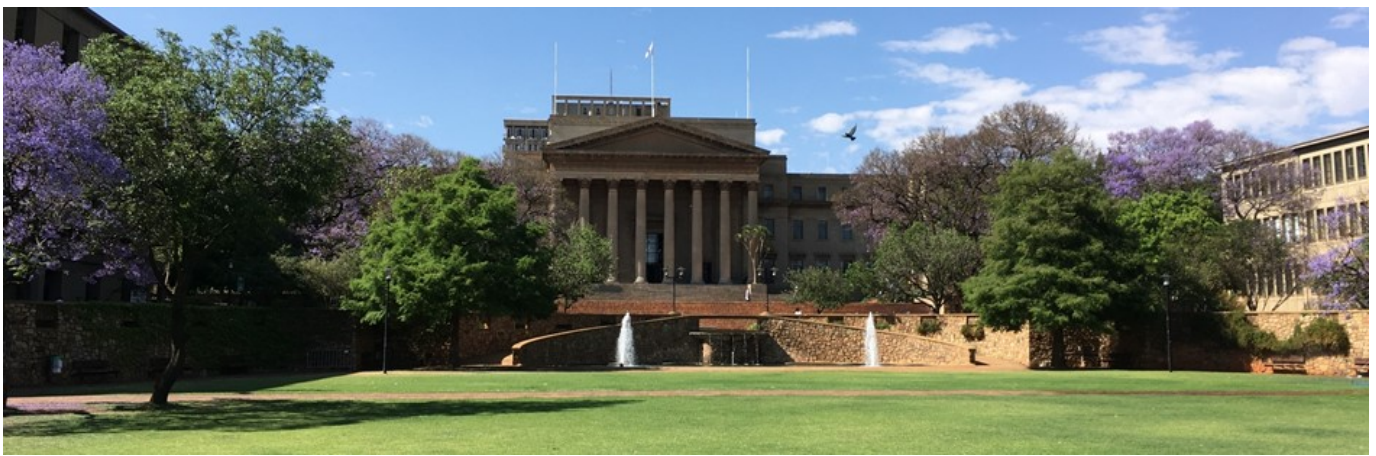
Figure 1: Main building of the University of the Witwatersrand, Johannesburg, South Africa.
